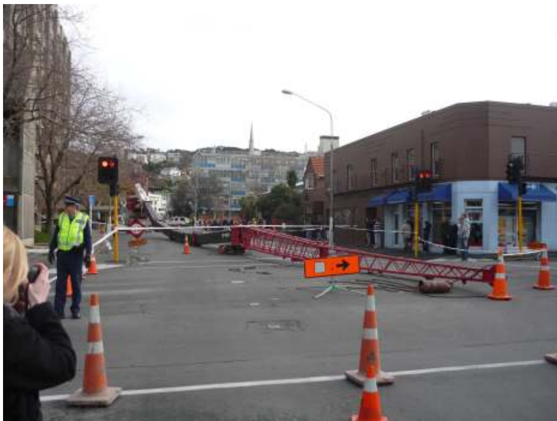
The fallen crane's jib lies across the intersection. The hospital building is on the left.
