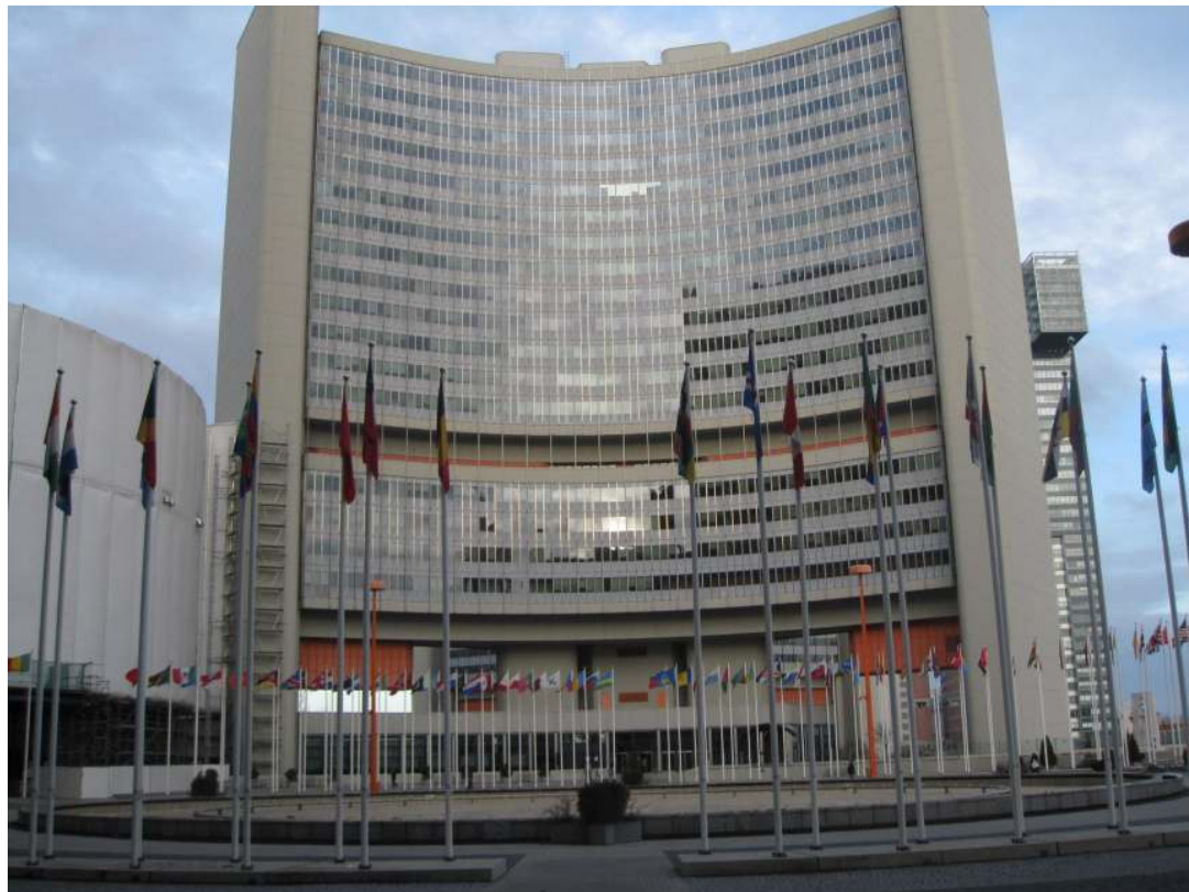
The Vienna International Centre (VIC), in Austria where Colin attended the International Symposium on Standards, Applications and Quality Assurance in Medical Radiation Dosimetry. Photo credit: Colin Rooney
